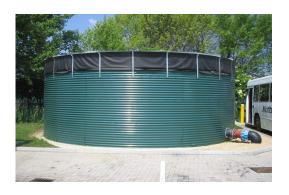
Circular corrugated sectional galvanised steel water storage tank complete with either standard PVC liner (10 year warranty) shaded liner (15 year warranty) or butyl and potable water liners.
